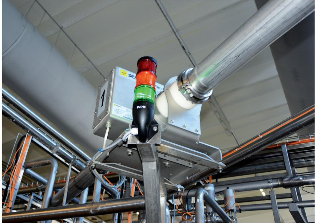
Sesotec metal detector P-SCAN RG installed in a horizontal conveyance pipeline
